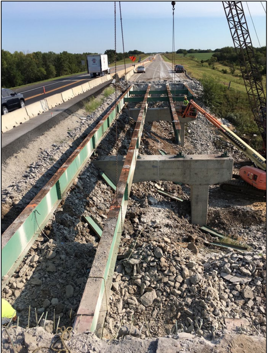
Crews remove a bridge along the Kansas Turnpike in Osage County.
