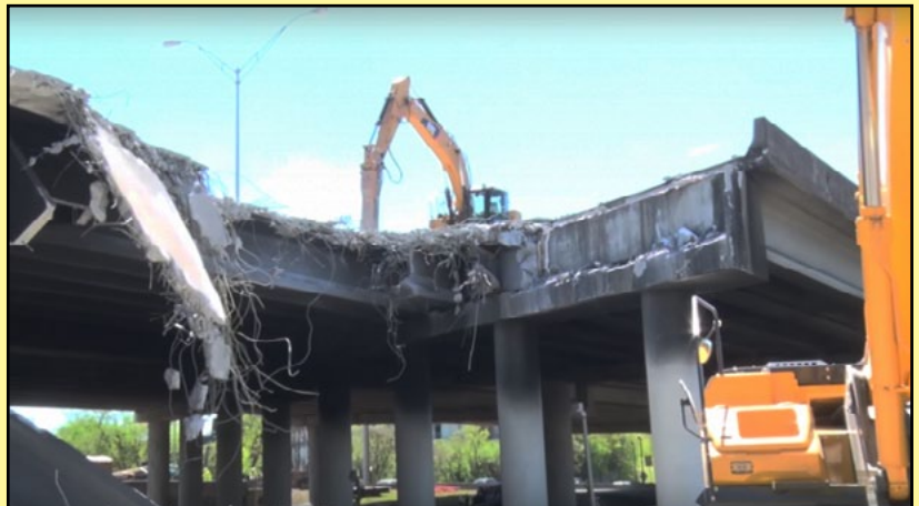
Demolition of I-85 after fire (Photo courtesy of Better Roads).
