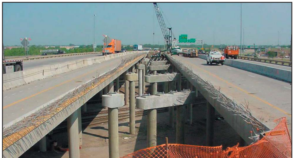
I-135 bridge widening in Wichita will continue this year.
