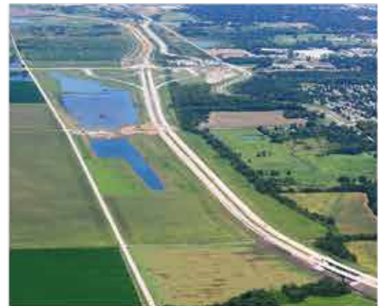
Construction of the SLT was essentially completed in November 2016.
