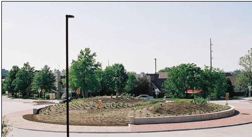
Overland Park, Kansas – 110 th Street at Lamar Avenue
