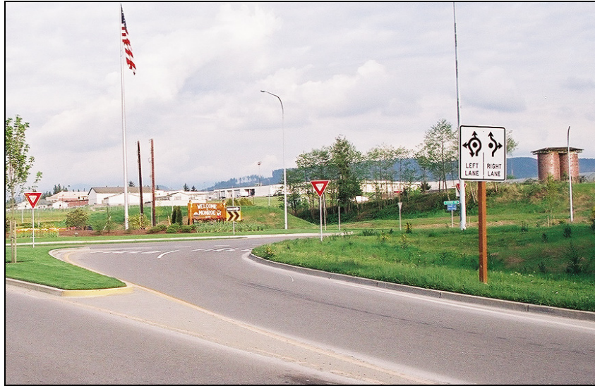
Exhibit 2-4 Approaching a Multilane Roundabout.
