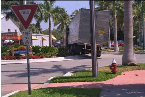
Example of roundabout not properly designed to accommodate large trucks
