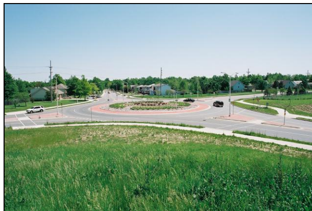
Roundabout, Olathe, Kansas
