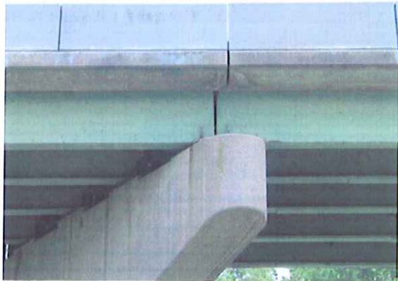
Photo 3: Example of open concrete joint used by bats
