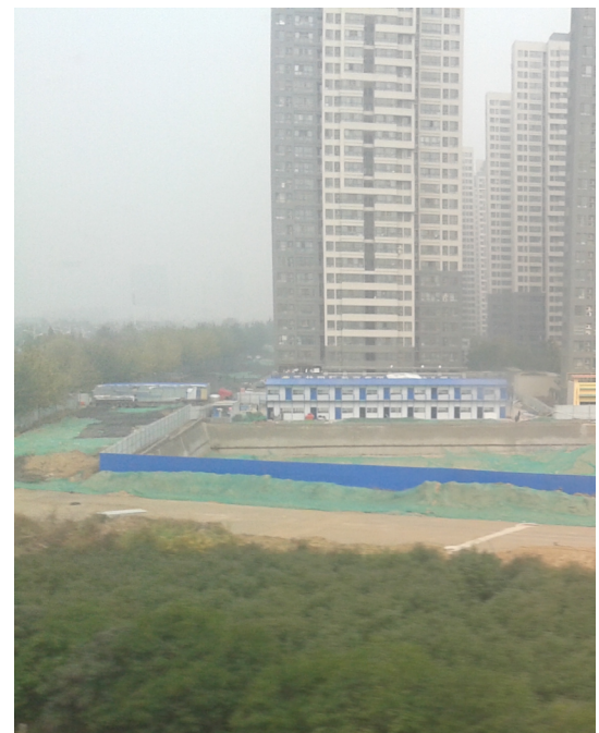
Plastic covering around the base of a new development.
