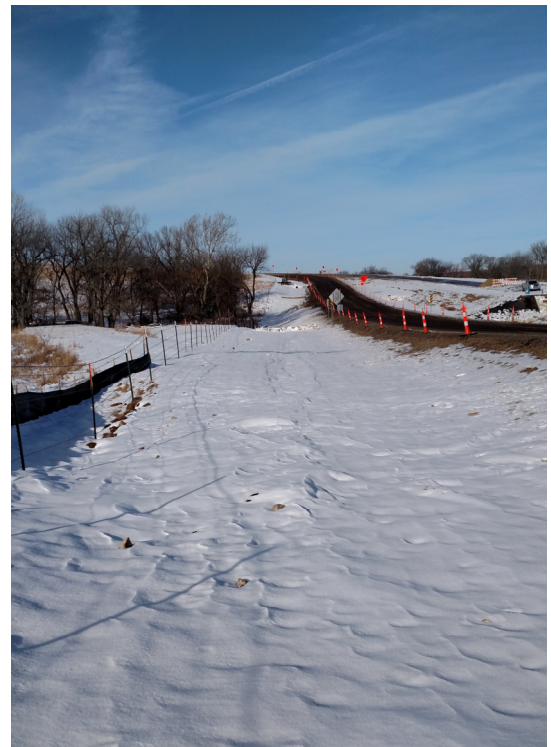
Temporarily stabilized project
