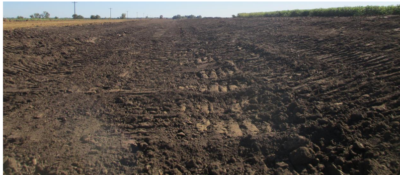
Soil after compaction. Notice the irregular chunky surface
