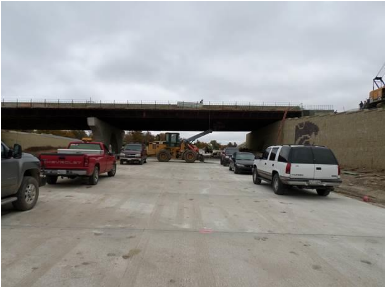
This is the new Miller Parkway/Davis Drive interchange bridge spanning K-18 which opened to unrestricted traffic today. (Photo taken: Tuesday, November 5, 2013)
