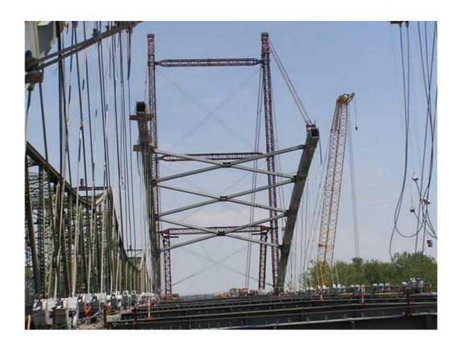
PROJECT UPDATE: The north side (left side in photo above taken on June 6) of the arch span section was successfully connected on Wednesday, June 13 at approximately 10:00 a.m. Crews hoisted the piece beginning at 7:30 a.m. but due to a few minor delays, it was not fully connected until 10:00 a.m. The south side (right side in photo above) is scheduled for connection (see below for more information) this Friday, June 15 between 7:15 a.m. and 7:30 a.m., pending any unforeseen delays.
