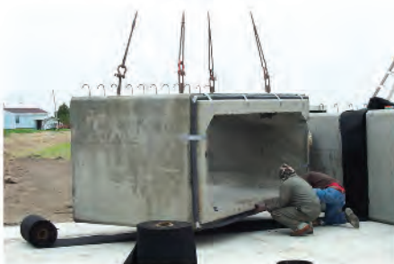
Workers place a box bridge along a county road on a Finney County project.
