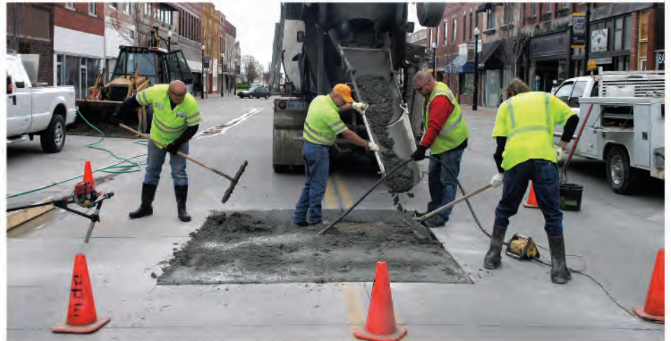
City workers make repairs on Main Street in Parsons.
