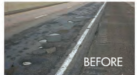
A section of westbound I-70 west of Ruleton in Sherman County before and after a preservation project to rebuild both eastbound and westbound lanes of I-70 from the Colorado/Kansas border east 12 miles.
