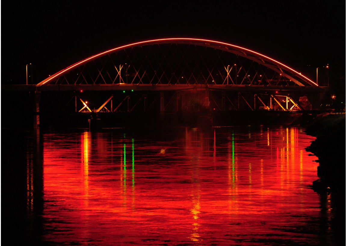
The Amelia Earhart Memorial Bridge was lit in orange last year as part of National Work Zone Awareness Week.
