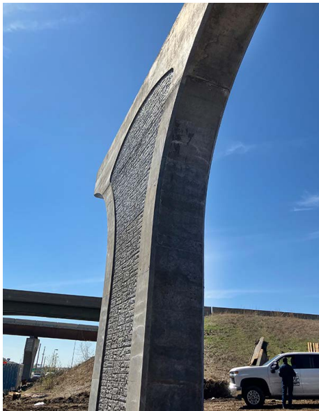
A new pier (above) and dirt work (right) are in progress as part of the westbound K-96 to southbound I-135 two-lane flyover being constructed in this phase of the North Junction project in Wichita. Photos by J.B. Wilson
