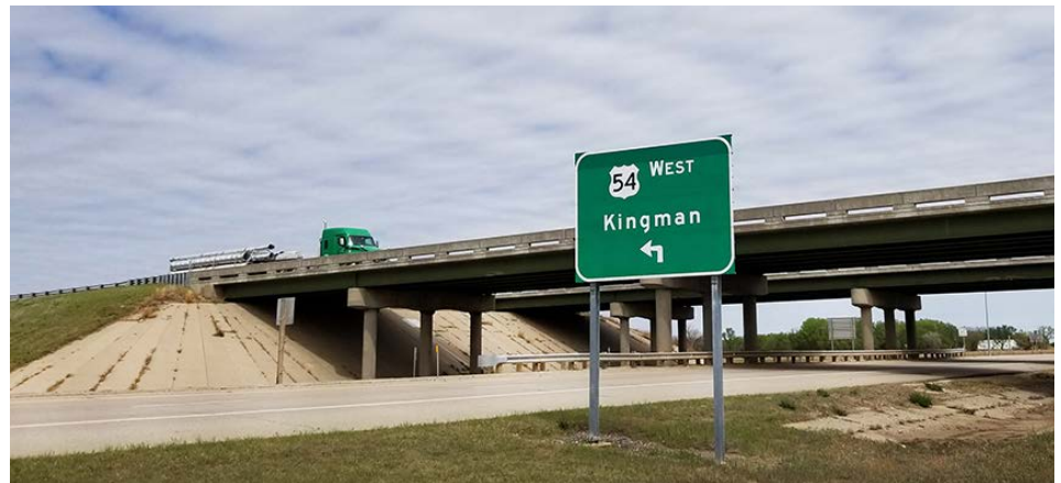
Eastbound U.S. 54/400 over the interchange at K-14. The bridge decks are part of a $36 million project. Photos by Tim Potter
