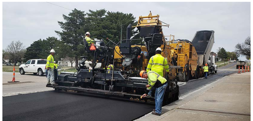
Construction in full swing Above, Daryl Dougherty (right), Engineering Technician Supervisor, Phillipsburg, inspects the overlay on the U.S. 283 project in Norton. Left, crews mill on U.S. 281 north of Russell in preparation for the new pavement. Photos by Lisa Mussman and Dean Jay, Hays
