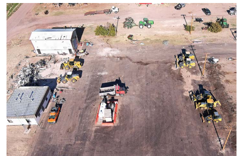
Pictured at top, the new buildings and equipment bays at the Sharon Springs Subarea. Above, a bird's-eye view of the damage caused by the tornado on April 22, 2022. Courtesy photos
