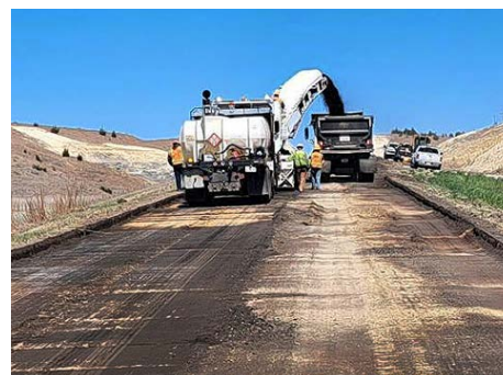
Construction in full swing Above, Daryl Dougherty (right), Engineering Technician Supervisor, Phillipsburg, inspects the overlay on the U.S. 283 project in Norton. Left, crews mill on U.S. 281 north of Russell in preparation for the new pavement. Photos by Lisa Mussman and Dean Jay, Hays
